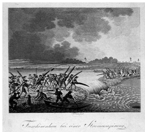
Figure 5. Constructing Faschinen .
